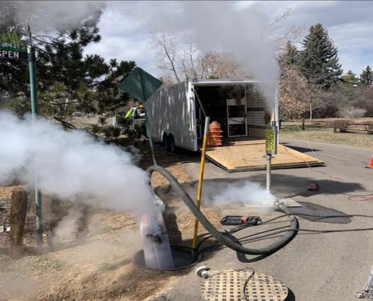
Steam cure; 3334' of 8" Pipe – 5 days to complete the lining work – Cost – Approx $200,000
