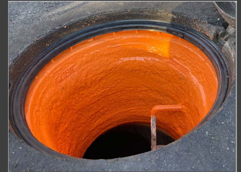
Chimney after Lining
