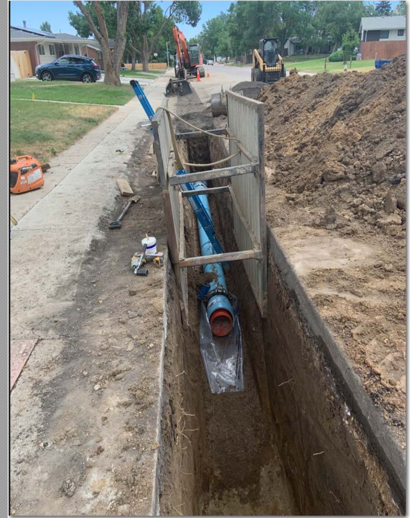
Example of Trench – pipe protection
