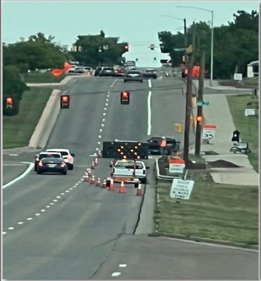
S. Kipling Pkwy at W. Fair Ave – Looking North
