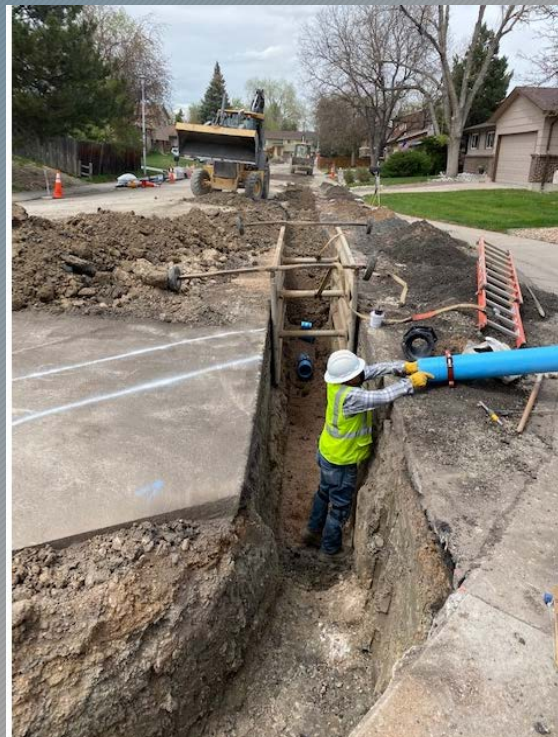
Flower Way 6" Water Trench
