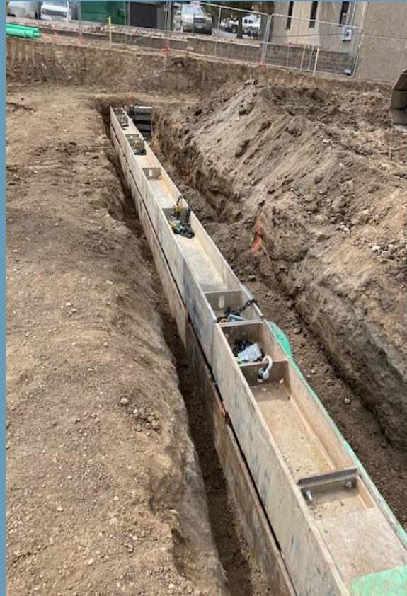
Hydraulic Support for Piling
