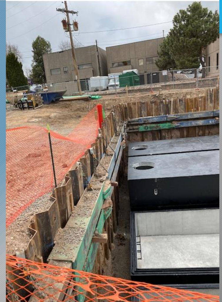
Overflow Tank Installation
