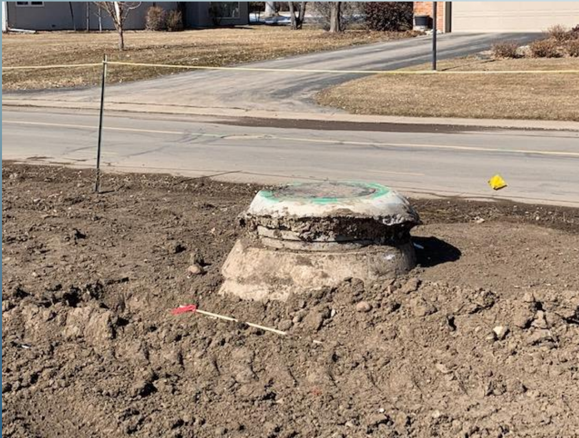
Manholes on B-Line to be lowered
