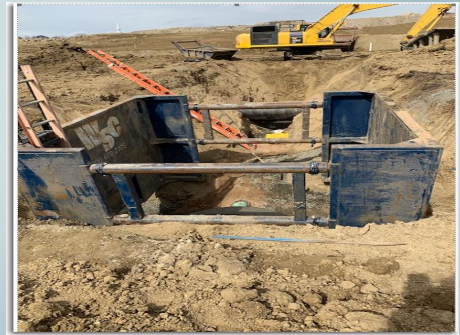
Laying New C-900 PVC Sewer Main Using Expansive Soil Backfill Requirements
