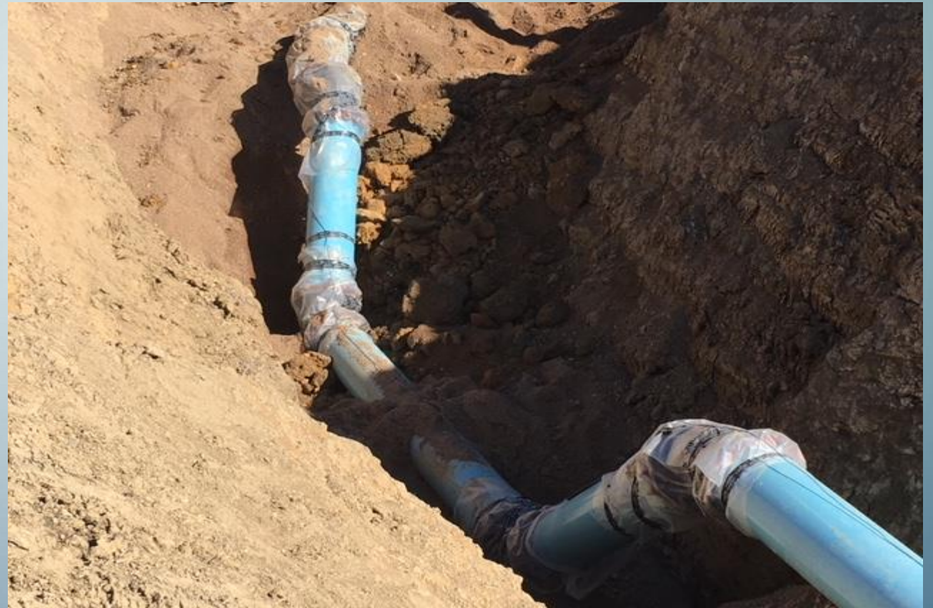
Water Main Lowering
