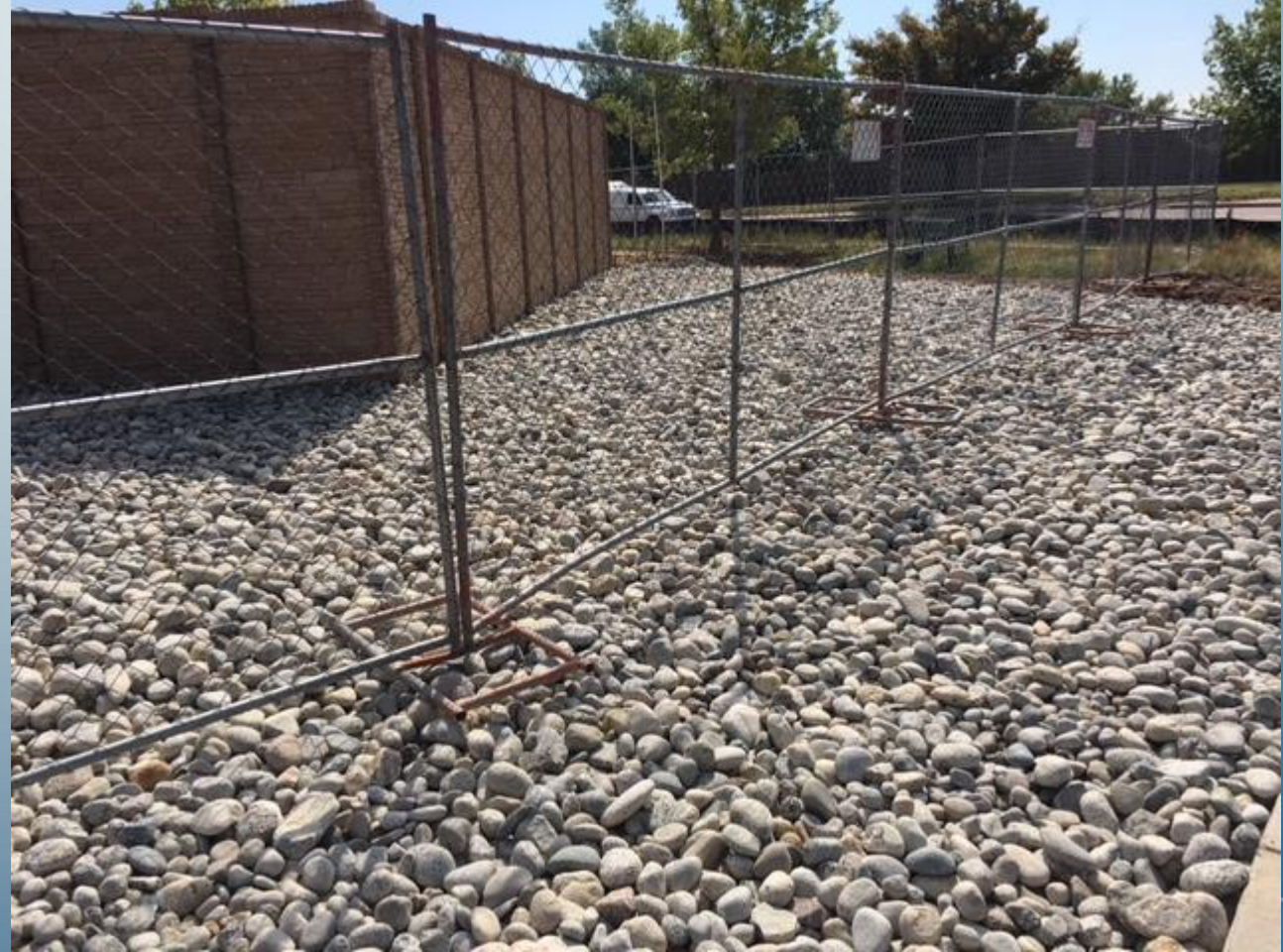
Fence/Wall on South Property Line
