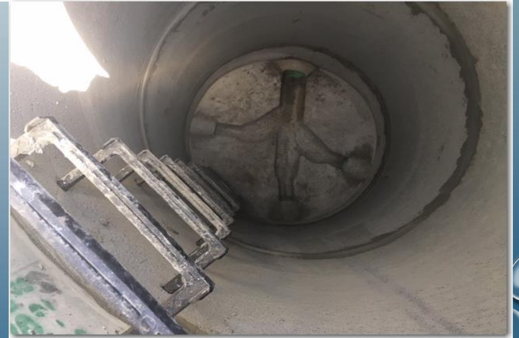
3-Way Service Connection to End Manhole
