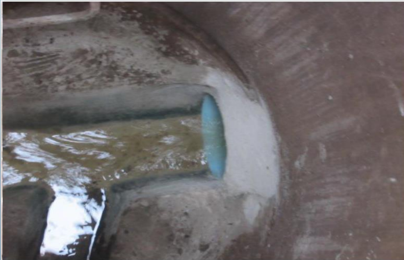
Picture 4- MH KV-17
