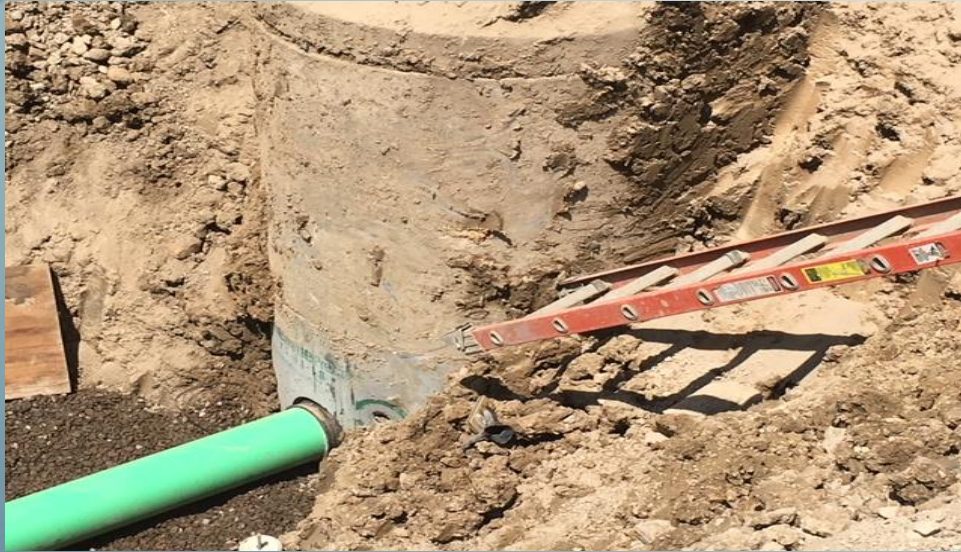
Connection to Existing Manhole
